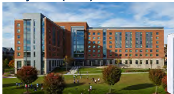
UMCP Frederick Hall, Maryland (USA)
